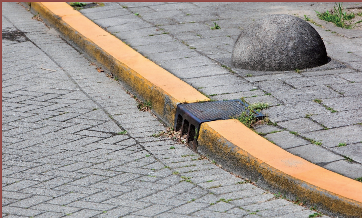
Figure #14 Example of yellow no parking curb. Source: Adobe Stock Images.
