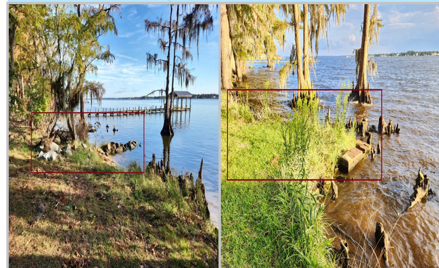
Example of installed groin. Source: Team picture on 10/26/2023
