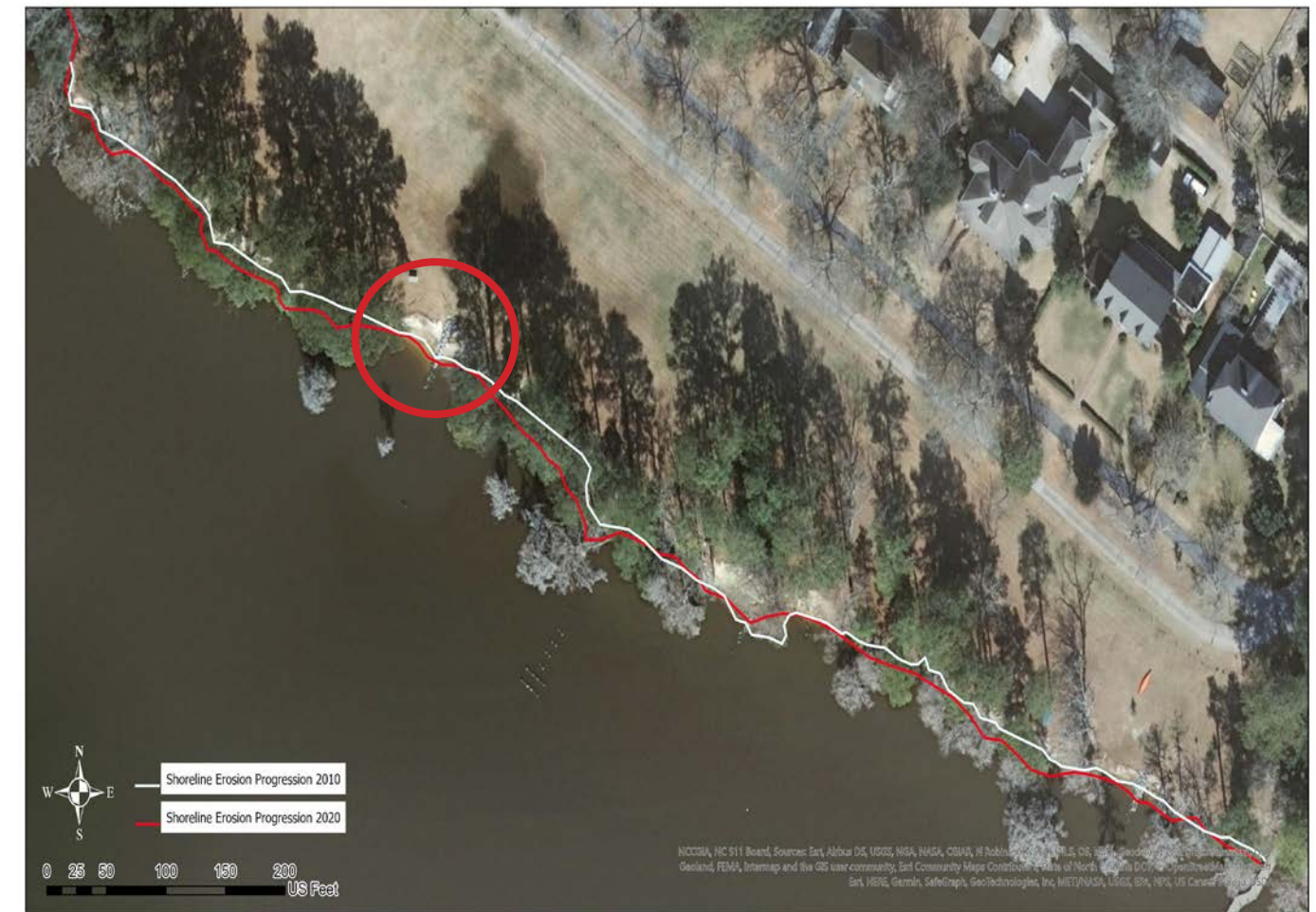
FIGURE 3 SHORELINE EROSION HISTORY Washington Park Site Erosion Within a 10 Year Span
