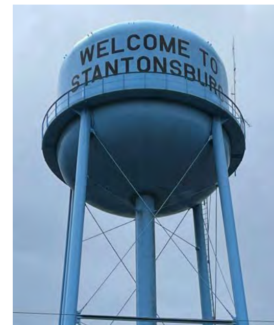
Figure 6. Stantonsburg water tower (image from https://www.townofstantonsburg.com/ )
