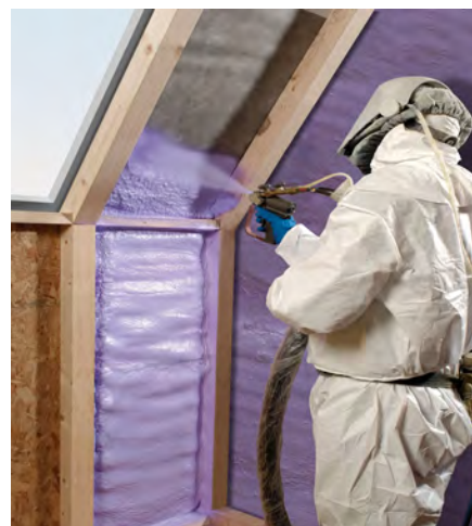
Photo 15. Foam Insulation
